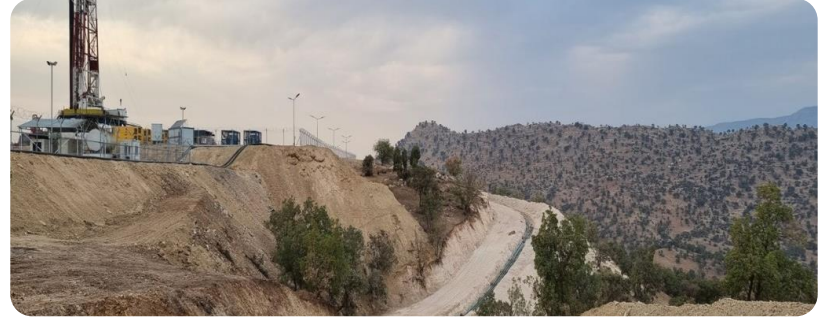
SH-16 & SH-17 flowline installation
