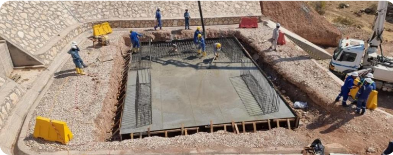
PF-1 flare knock out drum preparation
