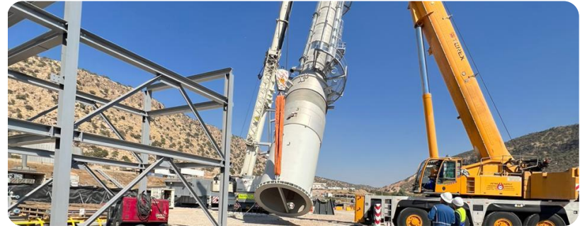
PF-1 stabiliser tower installation
